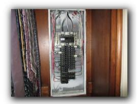
**Arc Fault Circuit Interrupter protection?** Inspector observed and tested arc fault interrupter breakers inside the electrical panel. No deficiencies noted. See Texas Real Estate Commission promulgated FORM OP-I, page 2, for information on AFCI and other safety provisions for homes.
