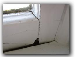
• Observed what appears to have been water intrusion\* on the interior sill at the window in master bedroom south window. Paint is peeling, chipping or sill is warped.
