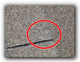
Nail head visible at south slope near the ridge. Recommend proper repair by a qualified roofing specialist.
