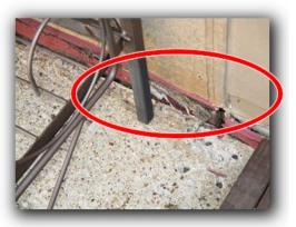
• Rear entry door wood trim is water damaged and deteriorating. Recommend replacing any damaged portions, re-painting and re-sealing trim to prevent further deterioration.
