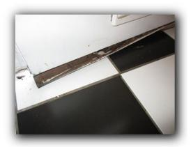
Wood trim is water damaged or rotted and deteriorating at the abandoned rear entry door.
