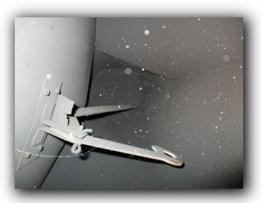
Rain cap at top of chimney has been damaged, and may be restricting exit of smoke from the fireplace. Any evaluation or subsequent repairs should be performed by a certified chimney technician.
