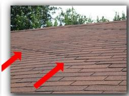
There are tree limbs and/or shrubs in direct contact with the roof at east side. All trees should be trimmed back 3 to 5 feet from the structure. When trees are close to the house, their limbs should never touch the building, or serious damage can result.
