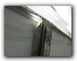
Operator on west side overhead garage door is in need of repair. Closing the overhead garage door operator requires holding the button for the full close cycle. When the button is released during close cycle, the door reverses itself.
