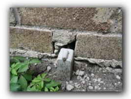
Observed vegetation/foliage in direct contact with the exterior of the structure. All plants and shrubs should be trimmed 3 to 5 inches away from the structure, to minimize wood rot and potential insect damage in siding and trim.
