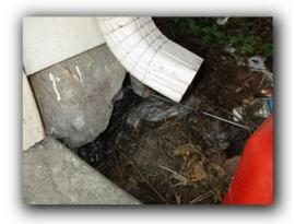
**<u>FYI: Water/Rain Management:</u>** Gutters and downspouts, efficiently diverting water away from the house, is one of the most important factors in preserving the integrity and extending the life of the foundation. Client should monitor site drainage conditions over time, especially during rainy weather, and have improvements made, as needed, by a qualified foundation repair or landscaping professional, if drainage anomalies develop.
