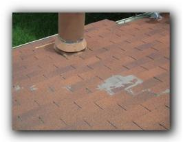
Bruising and scraping from previous limb contact observed at shingles at west end of roof.
