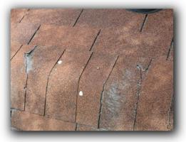
Shingle rows have not been properly staggered, so that diagonal shingle tab corners appear
