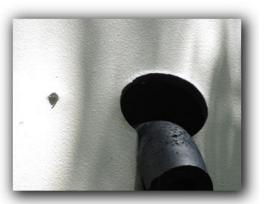
Observed gap in the brick and mortar at the east side, where electrical cable exits the house for service to the tool shed. Recommend sealing gaps to prevent rodents or vermin from entering the wall cavities.
